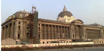
Sichuan Museum, Chengde, which was intact (except for a few cracks) during the earthquake. It was at the
